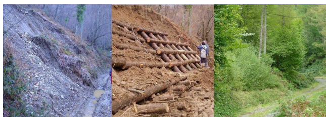
Landslide stabilisation in Forestry -P. Sangalli
