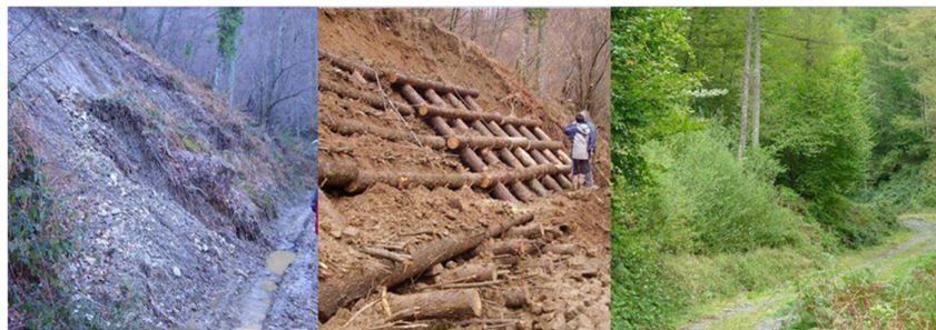
Slope stabilisation in Forestry -P. Sangalli
