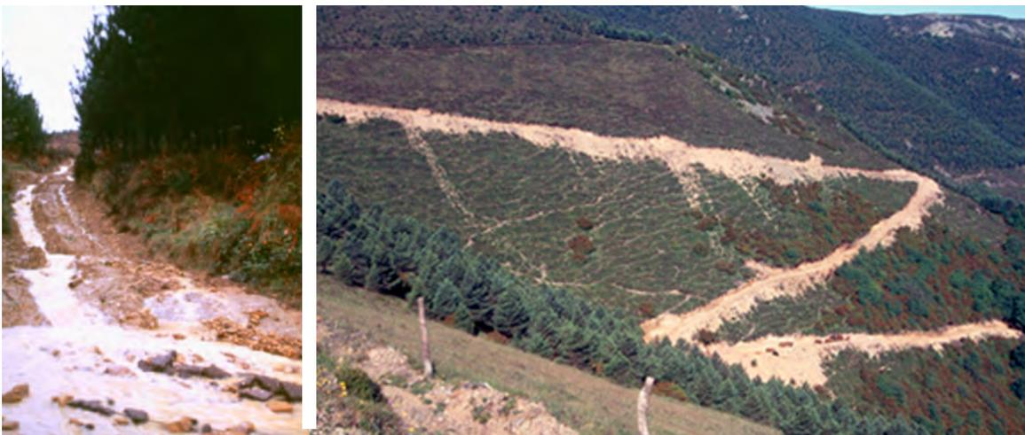
**Figure 10.** Poorly designed forest roads generating large amounts of run-off (Bizkaia and Lugo, respectively, Spain).
