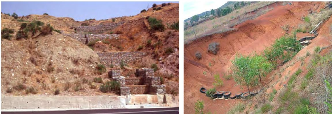
**Figure 18.** Constructions of a series of dams and other actions for preventing the gully increasing in size.
