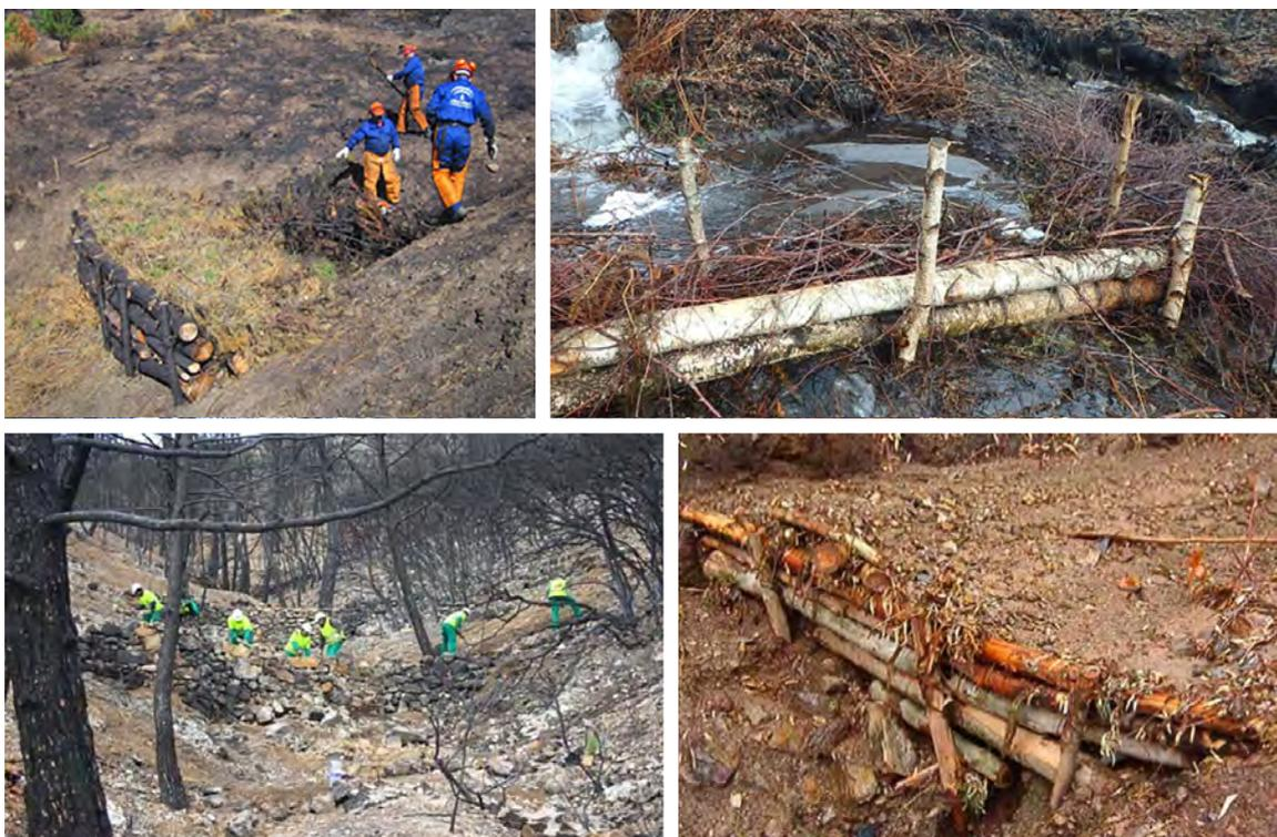
**Figure 20.** Small dry dams installed to retain sediments, flooding mitigation and slope stabilization. Photos courtesy of CIF Lourizan (upper) and by Agustín Merino (lower)
