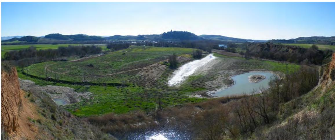
**Figure 2.** Restoration works on the Plantío meander (Arga River, Navarre), including different natural water retention measures, such as: reconnection of paleo-channels, creation of wetlands, plantation of forest patches with native species (local genetics) and improvement of habitats by increasing the topographical heterogeneity and the ecohydraulic complexity of the project area.
