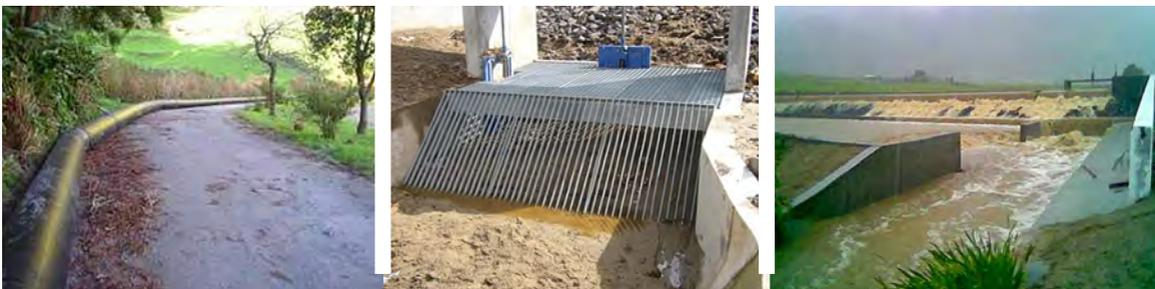
**Figure 9.** Water and nutrients by-pass with a retention basin in Sete Cidades lake, Azores (Source: courtesy of D. Pacheco).
