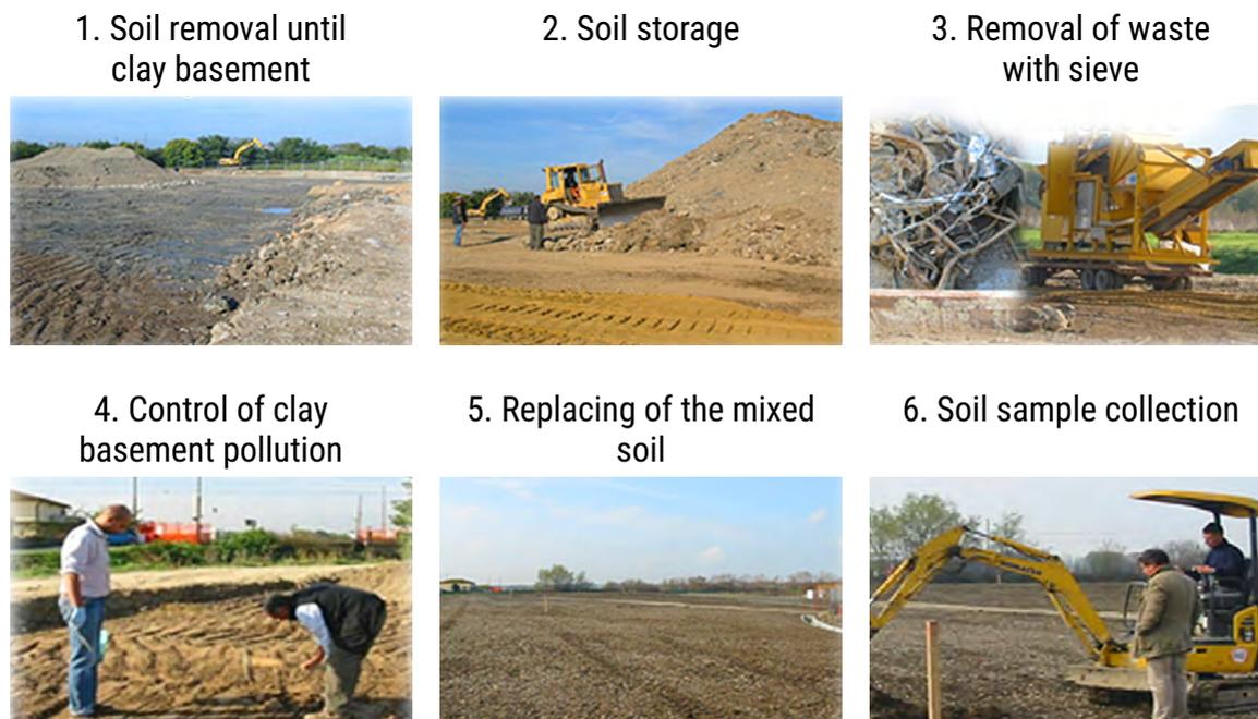
**Figure 1.** On April 2007, the polluted field was divided in five plots and in each plot the soil was removed until clay basement, the bulky wastes were removed manually and by sieving and, after mixing, the soil was replacing in the same plots.
